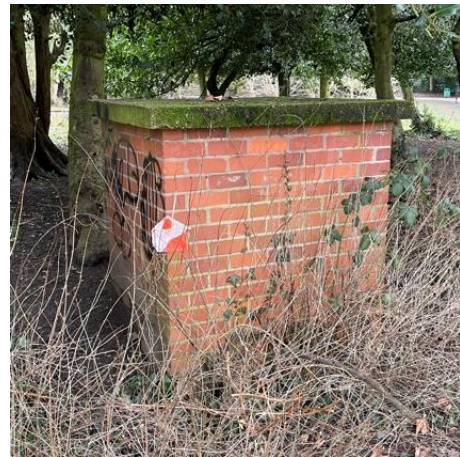
11. Building, NW corner: ESE
