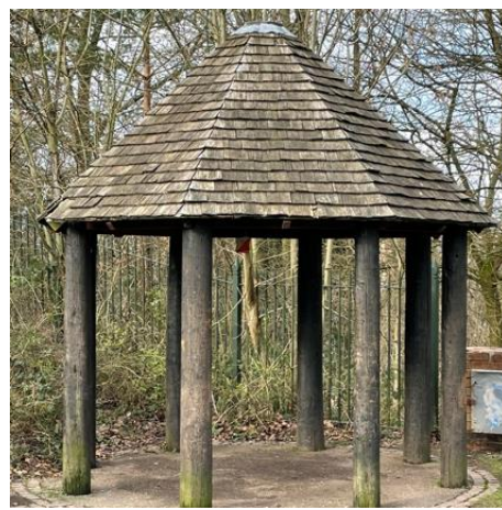
Finish. Building: NW
