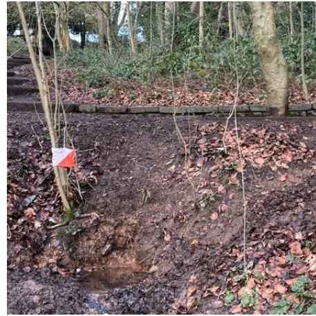
13. Wet ditch, N end: N
